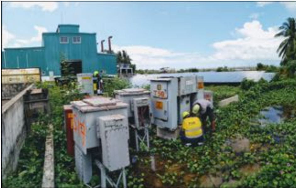
Photo 5 – Sampling Transformer Oil for PCBs
