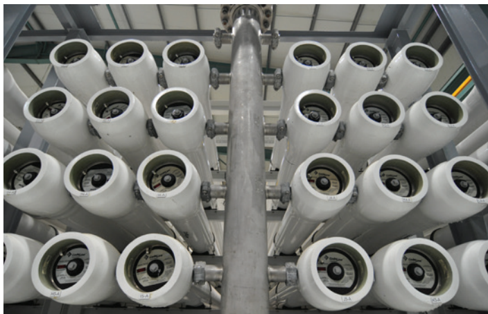
Figure 12 Superduplex piping in a Seawater Reverse Osmosis desalination plant [Photo courtesy of Rolled Alloys]
