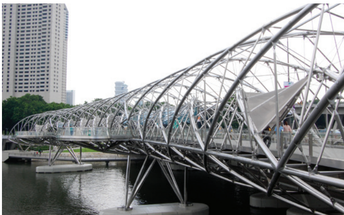
Figure 11 Marina Bay Bridge in Singapore constructed entirely of 2205 duplex stainless steel [Courtesy of Outokumpu Stainless AB]
